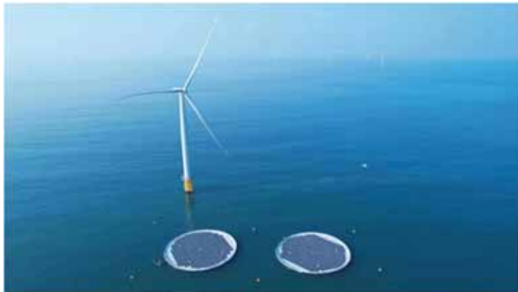
Combined floating solar and offshore wind farm in Shandong coast : SPIC
